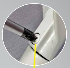
Use a phillips screw driver to loosen the set screw and pull off the window handle.
