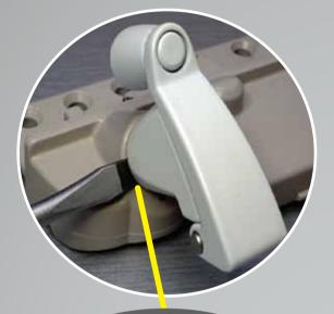
Insert a flat screw driver between the housing and the handle, gently pry off the window handle IF THERE IS A SET SCREW
