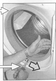
install spring clamp, carefully pull spring to right & put clamp into right side gasket notch.
