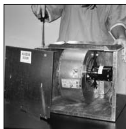
3. Install optional TDA panel and four screws.
