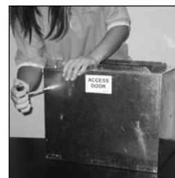
4. Re-install access panel and screws.
