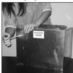
1. Discard grille and remove access panel screws.
