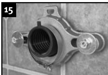
Install the gear clamp with the screw head at the bottom, but do not tighten.
