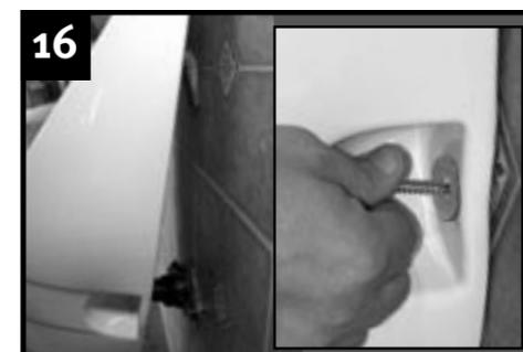
Hang the bowl, inserting tailpipe into bushing, then install anchor screws with washers. Tighten flange bolts and gear clamp.
