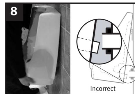
Hang the bowl on the bracket and check tail pipe alignment, then remove the bowl and adjust the bracket as needed.
