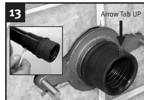
Apply lubricant to the outside of the rubber bushing and ribbed inside area. Insert the tube and bushing with the arrow tab at the top. Lube tailpipe of housing.
