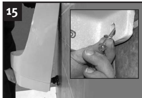
Hang the bowl, inserting tailpipe into bushing, then install anchor screws with washers.
