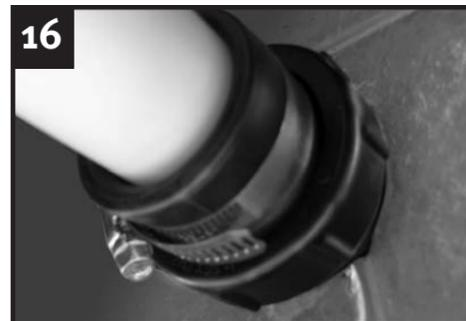
Tighten the compression nut and gear clamp.
