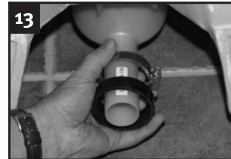
Place the gear clamp and compression nut onto the housing tailpipe. Apply lubricant to the tailpipe.
