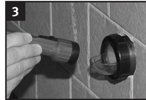
Use a flashlight to check pitch/slope. There should be no water present in the inspection disc or nipple. Remove compression nut after inspection.
