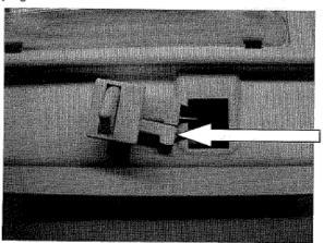
Rotate red with white stripe wire 180 degrees and plug into new light switch
